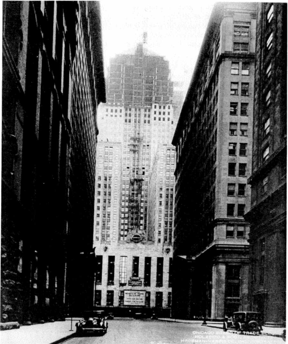
The Chicago Board of Trade Building under construction in November 1929.
